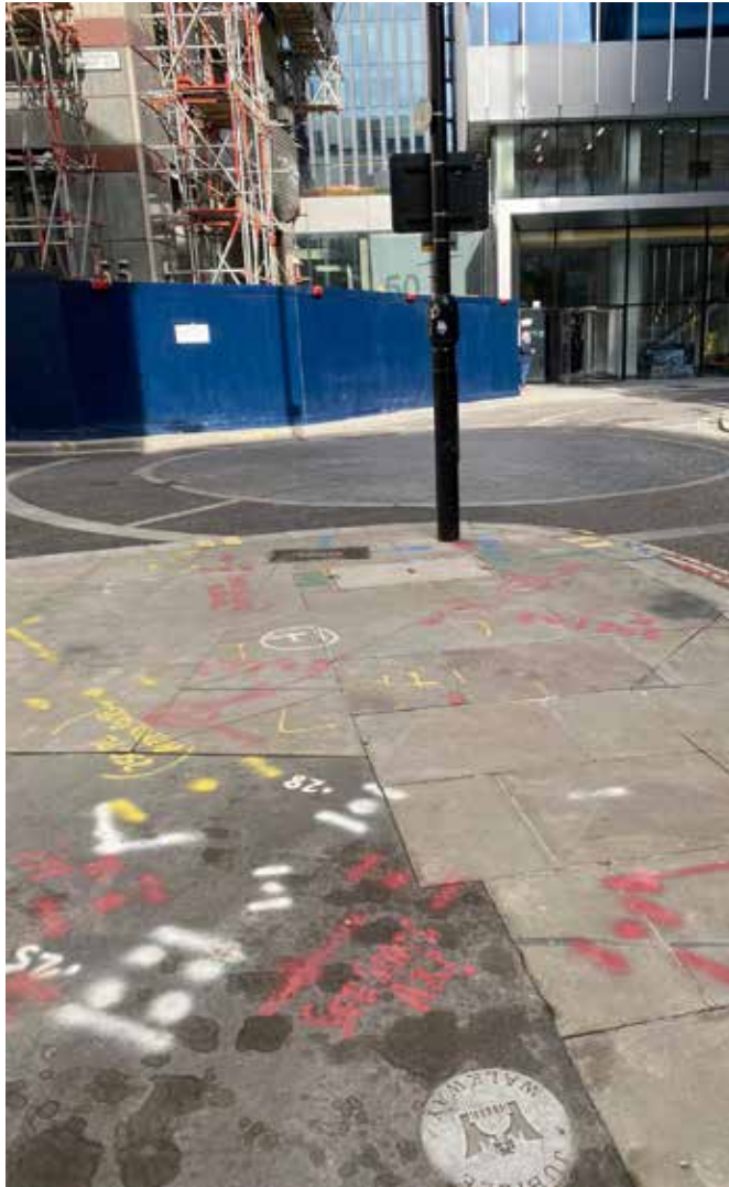
Trial hole location - T1 Basinghall Street
