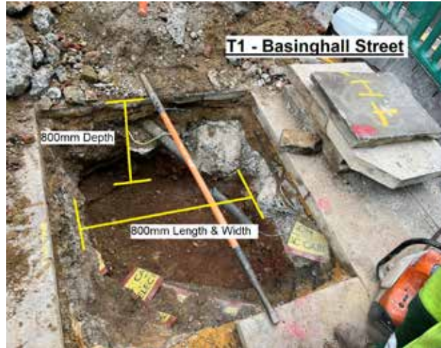
Trial hole excavation
